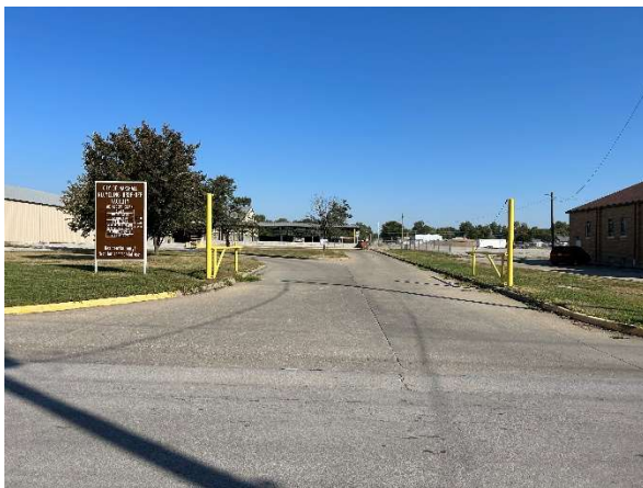
Entrance to recycling drop-off facility
