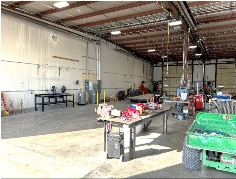
New Maintenance Shop
