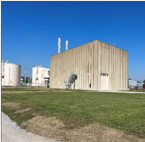
Units #10 and #11 Building
